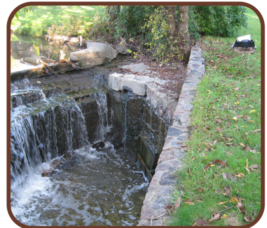
Danvers Pond dam prior to restoration
